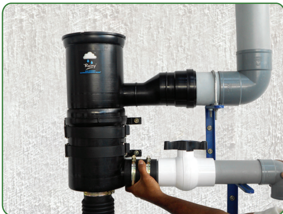
Fix bypass valve with suitable clamps and fixtures
