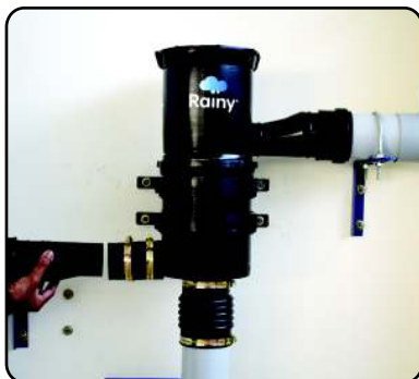
Insert adapter into the bush
